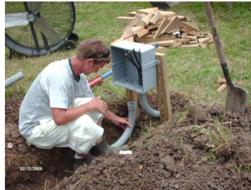
Step 5: Connect Conduit and Wiring
