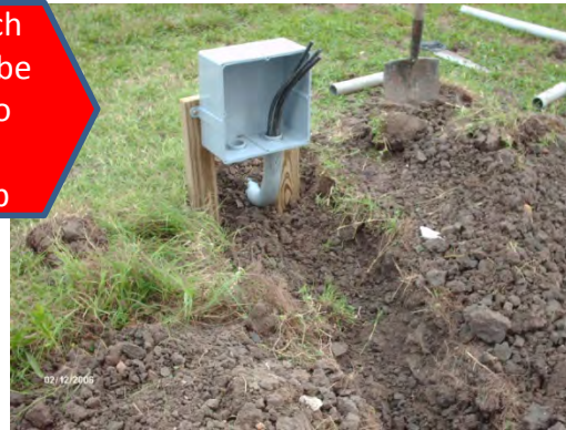
Step 2: Install Electric Box on Wooden Post
