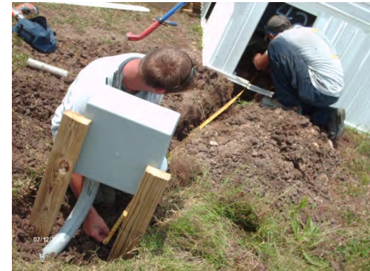
Step 3: Measure for Wiring
