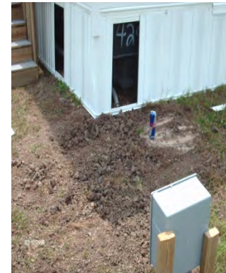
Step 6: Fill in the Trench and Secure Conduit Under Unit
