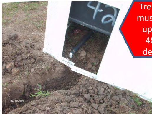
Step 1: Dig up to a Forty-Eight Inch (48") Trench from Unit to Electrical Box Location
